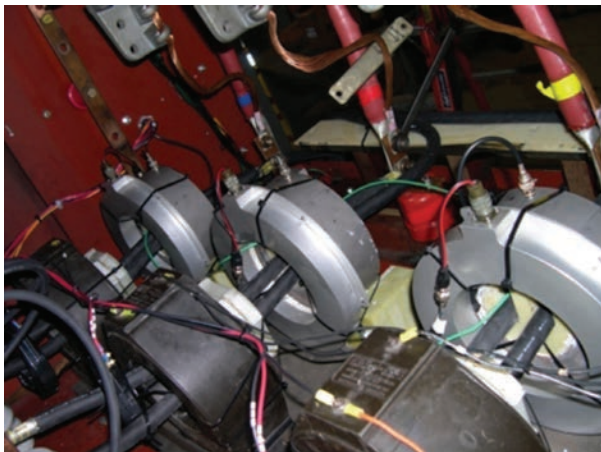
FIGURE 4: Photo inside motor termination vault. One HSCT is installed on each phase of power leads to the motor. Note: The HSCTs need to sense current in both conductors of each phase, so the MSIM system works with externally-terminated wye (star) connected stators, but not with internally-terminated or delta connected stators.
