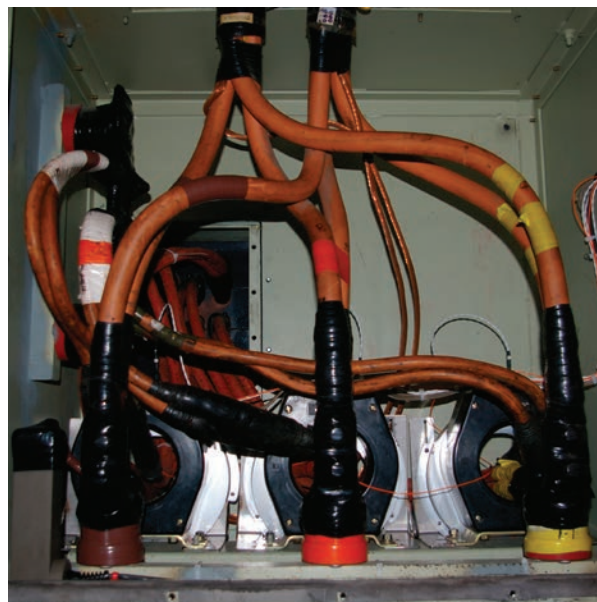
FIGURE 5: Field installation at a power generating station. The aluminum-cased HSCT transducers are behind the normal protection CT transducers (with brown molded plastic cases) in this photo.
