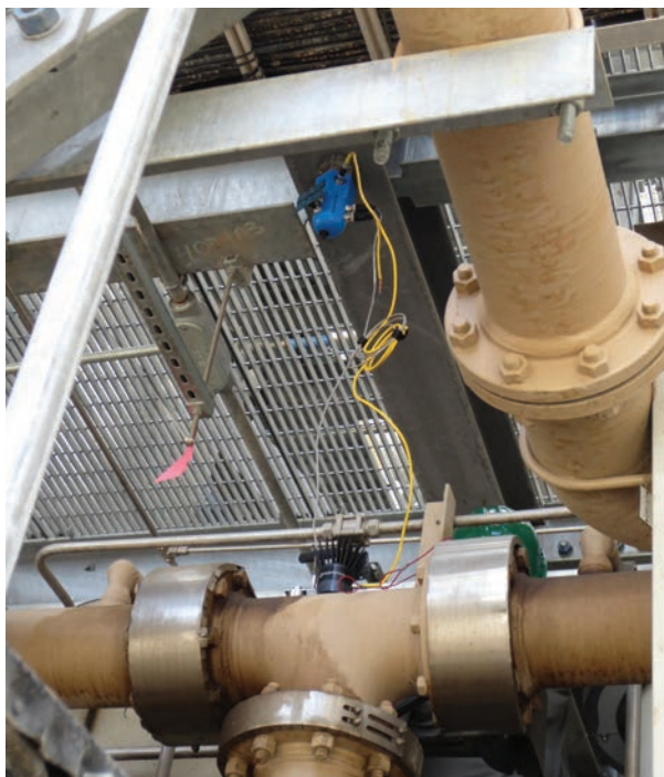
FIGURE 2: Hot Boiler Feedwater Line. In this example, the wSIM was hanging upside down from the overhead structure and the Power Puck was attached on top of the piping tee at the bottom of the photo.
