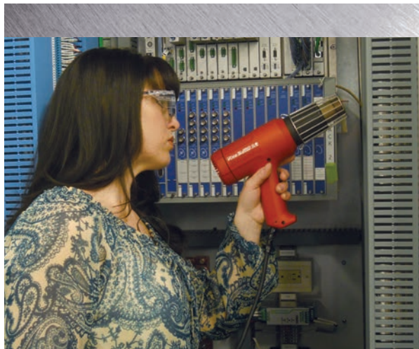
Projects Quality Coordinator Pam Litka shrinks tubing over wiring labels.
