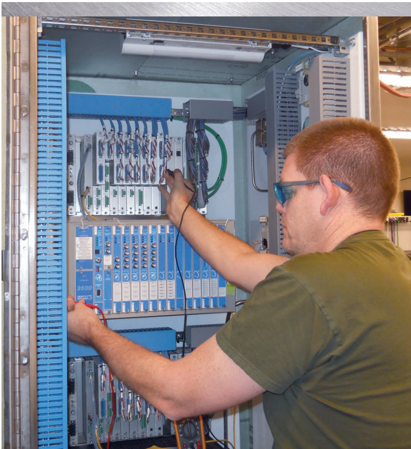
Manufacturing Technician Scott Smith performs power-off point-to-point continuity check.
